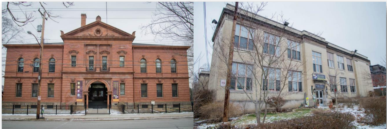
Figure 1: Environmental Charter School (left: Lower School, right: Upper School)
