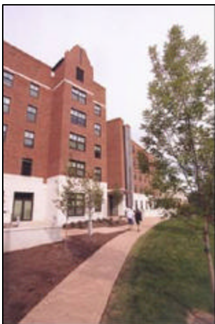
New House dormitory is silver LEED (Leadership in Energy & Environmental Design) certified.
