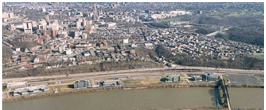
Right: Aerial view of PTC under construction (Source: URA, no date)
