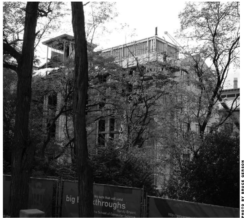
PHASE II OF THE DOHERTY HALL RENOVATION PROJECT CAN BE SEEN THROUGH THE TREES BETWEEN THE PURNELL CENTER AND THE DOHERTY HALL FRONT ENTRANCE.
