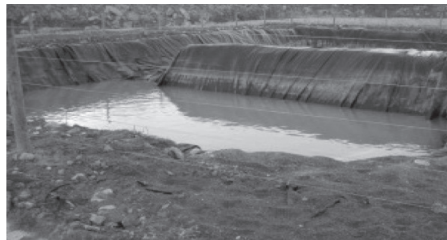
WASTEWATER, WHICH OFTEN INCLUDES TOXIC CHEMICALS THAT LUBRICATE DRILLING EQUIPMENT, OFTEN ENDS UP IN WASTEWATER PITS. BARKIN CITES INCIDENTS WHERE WATER FROM THESE HOLDING AREAS HAS CAUSED GROUND SURFACE CONTAMINATION.
