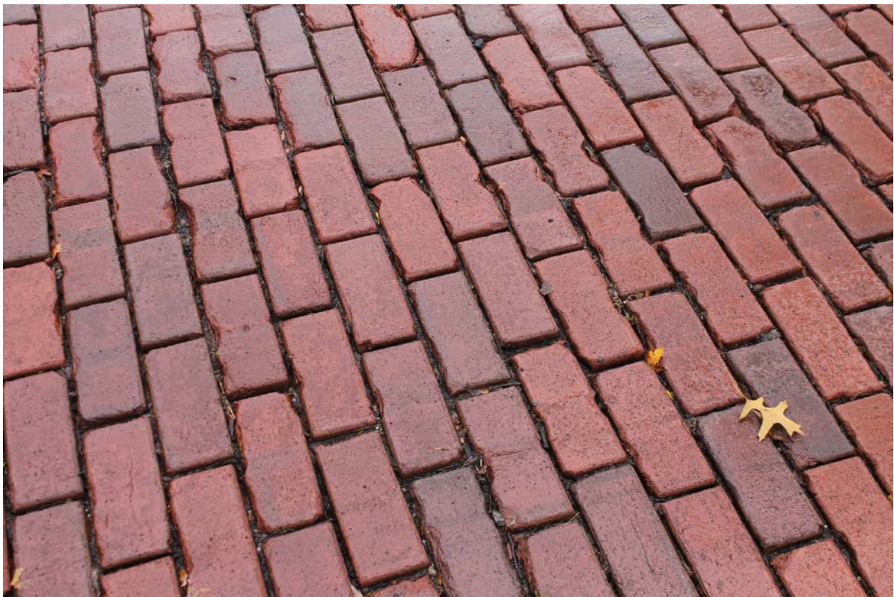
Image 3: Light chipping is expected and harmless in brick streets. Many argue these small imperfections add to the aesthetic of the street.
