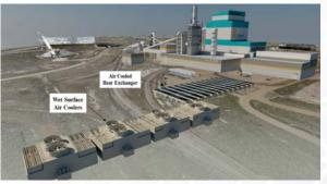
Figure 10. Proposed new hybrid heat rejection system
