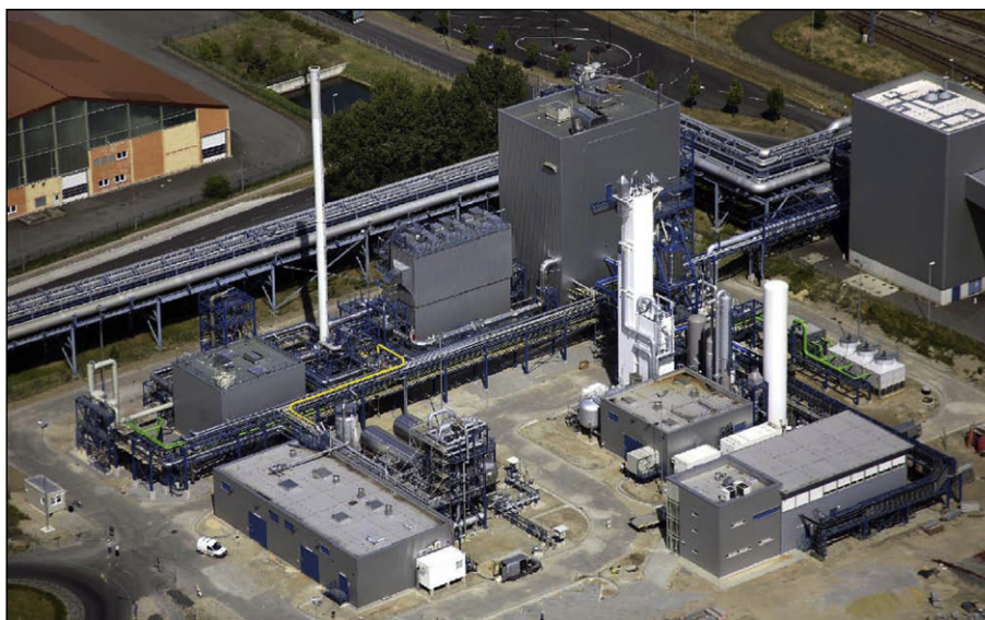
Fig. 23. Oxy-combustion pilot plant capturing CO 2 from the flue gas of a coal-fired boiler at the Schwarze Pumpe power station in Germany; Photo courtesy of Vattenfall.
