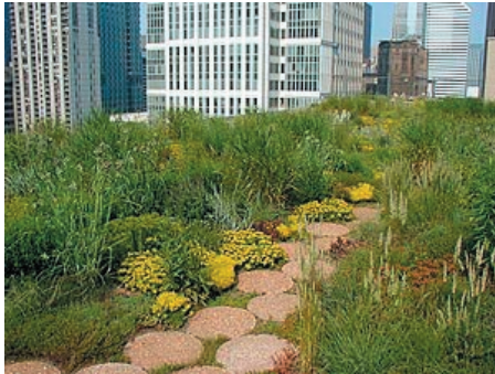
Example of a Living Roof on Chicago City Hall
