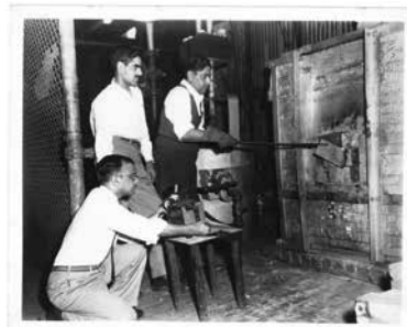
Ishwar Chand Modi is shown at center in this photo, which depicts students conducting experiments to assess the suitability of certain refractories for steel plant furnaces.
