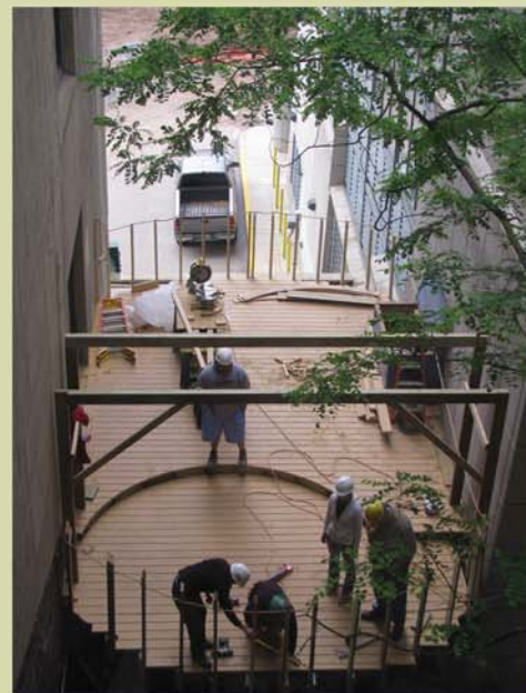
The work in progress
