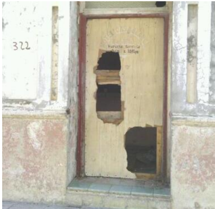
Entrance to Hotel Casa Blanca, on Loynaz and Merchán Streets.
