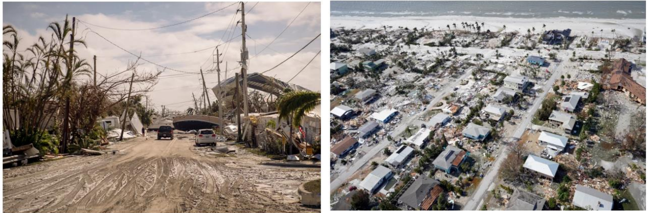
Figure 4.26. Left: Destruction from Hurricane Ian in Fort Myers, Florida with a surprising number of poles still standing. Photo by Hilary Swift of The New York Times . Right: Many homes in Fort Myers were destroyed. Photo by Wilfredo Lee of Associated Press . Photos accessed from: (Boston.com, 2022)
