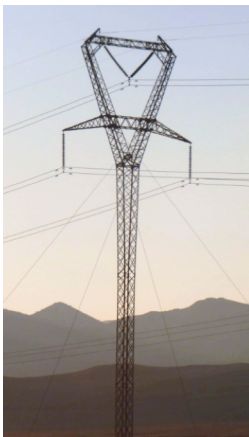
Figure 2: Example of a guyed transmission tower. Such towers can be less expensive but subject to “domino collapse.” Image from Wikimedia.
