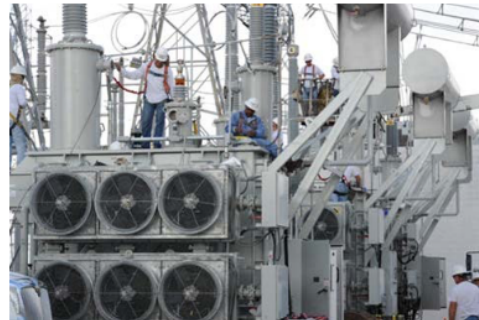
RecX in-grid deployment (Paul Wedig)
