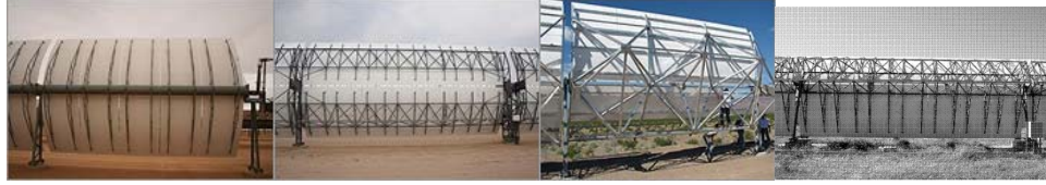
Figure 7 – SCA Metal Support Structure Designs.
