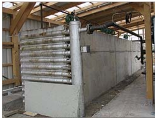
Figure 12 - Concrete Thermal Energy Storage System [59]
