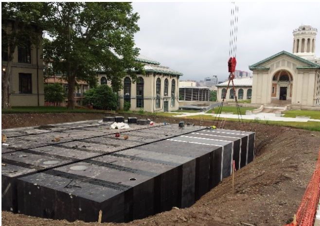
Stormwater Tank underneath The Mall
