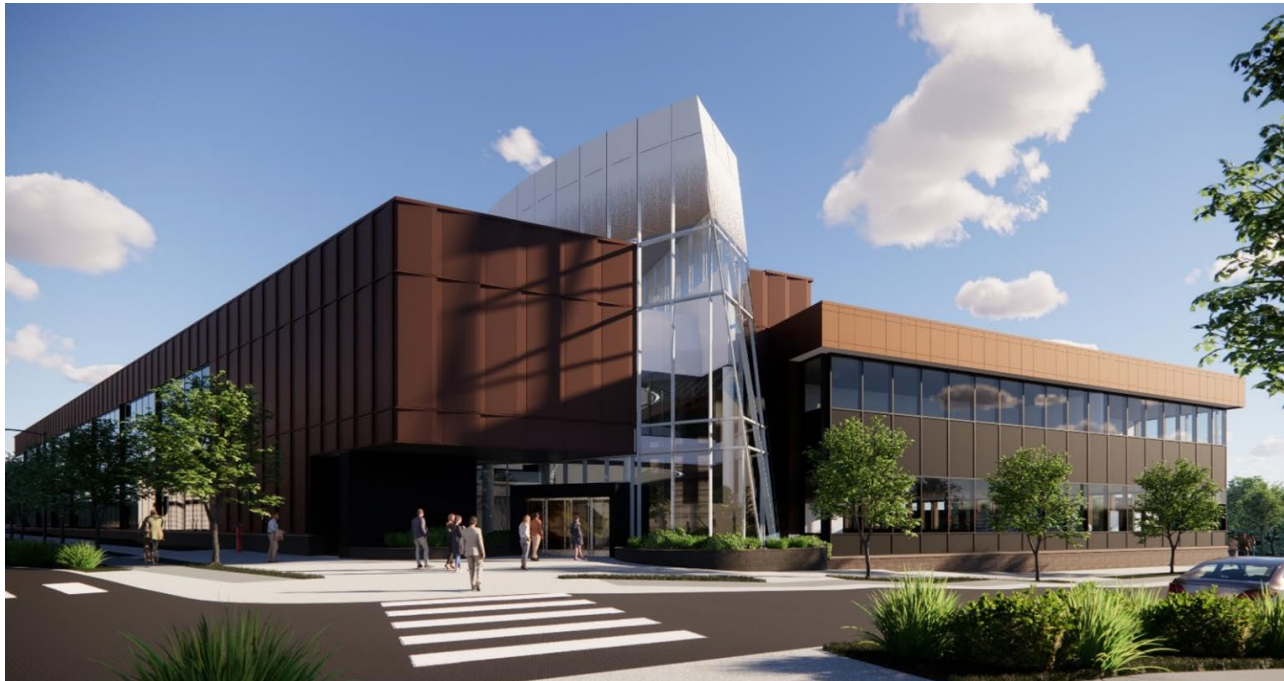
University of Pittsburgh Cell & Gene Facility – Beehive Street Entrance
