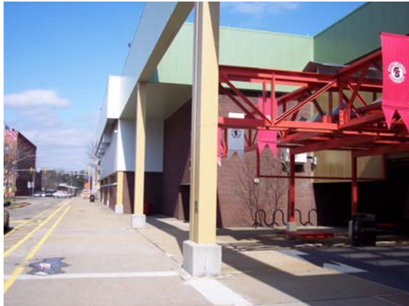
Photo Courtesy of 2009 Facility Assessment Report on Pittsburgh Public Schools Website
