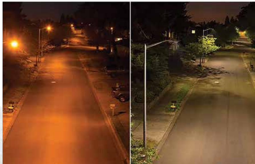
BEFORE AND AFTER: THE IMAGE ON THE LEFT SHOWS A NEIGHBORHOOD STREET LIT WITH SODIUM VAPOR STREETLIGHTS. ON THE RIGHT IS THE SAME STREET UNDER LED LIGHTING.
