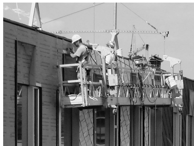
WORKERS PUT THE FINISHING TOUCHES ON THE GATES CENTER.
