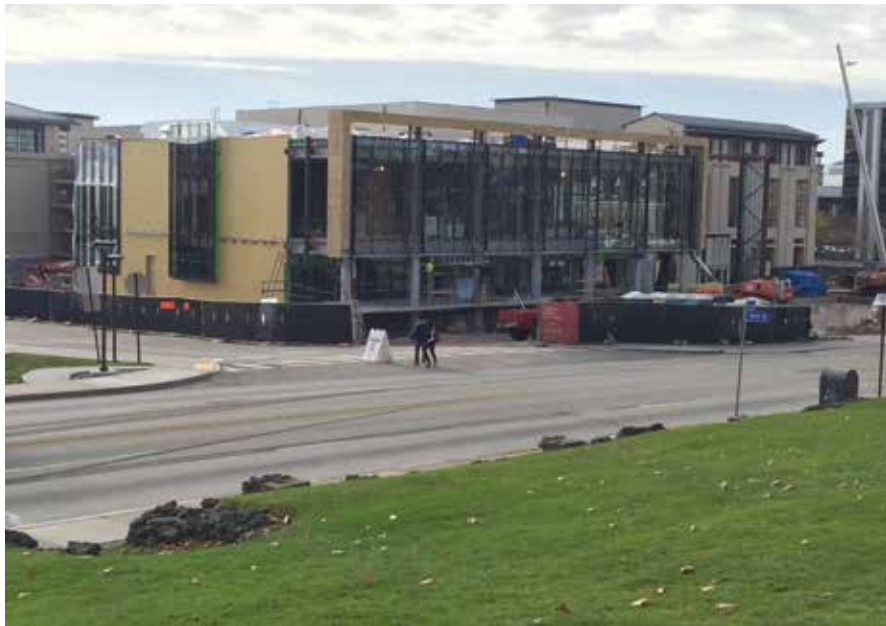
THE COHON CENTER ADDITION WILL BE COMPLETED THIS MAY.
