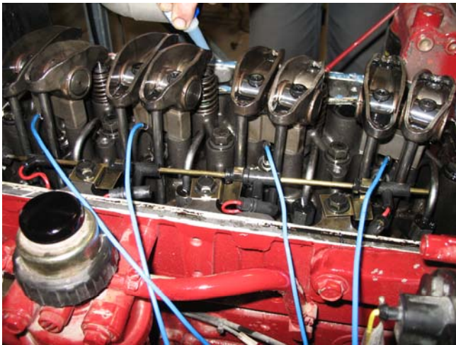
Figure 9. Pressure Sensor Installation (blue wires are data lines)
