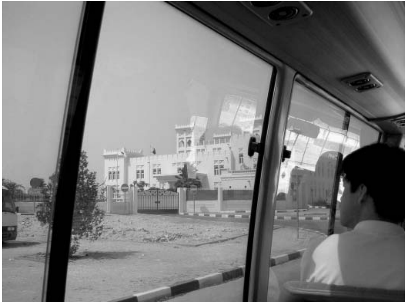
Approaching the Qatar Foundation offices, one of the completed buildings in Education City outside of Doha, Qatar, where Carnegie Mellon is building a new campus. Carnegie Mellon's building is still in the design stage. Photo: Chuck Thorpe.
