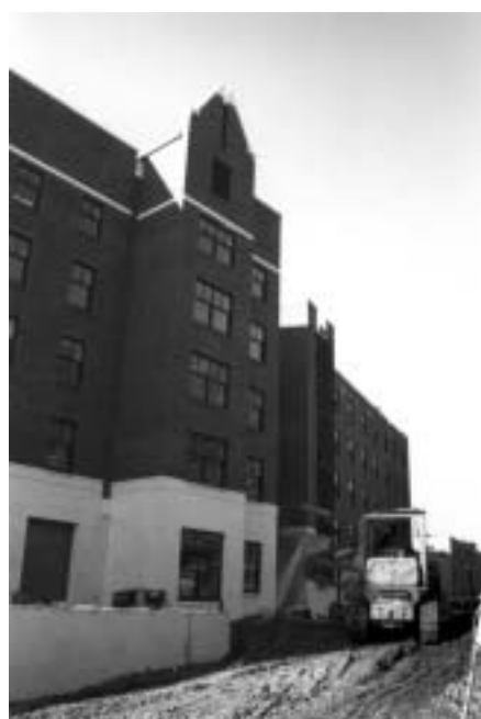
Grading the front of New House
