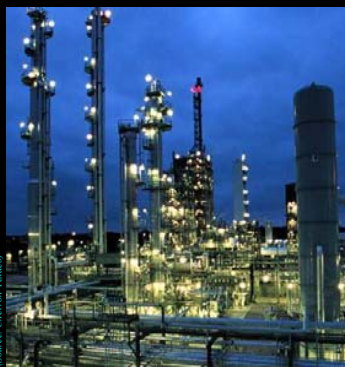
Petoche Gasification to Produce H 2 (Coffeyville, Kansas, USA)
