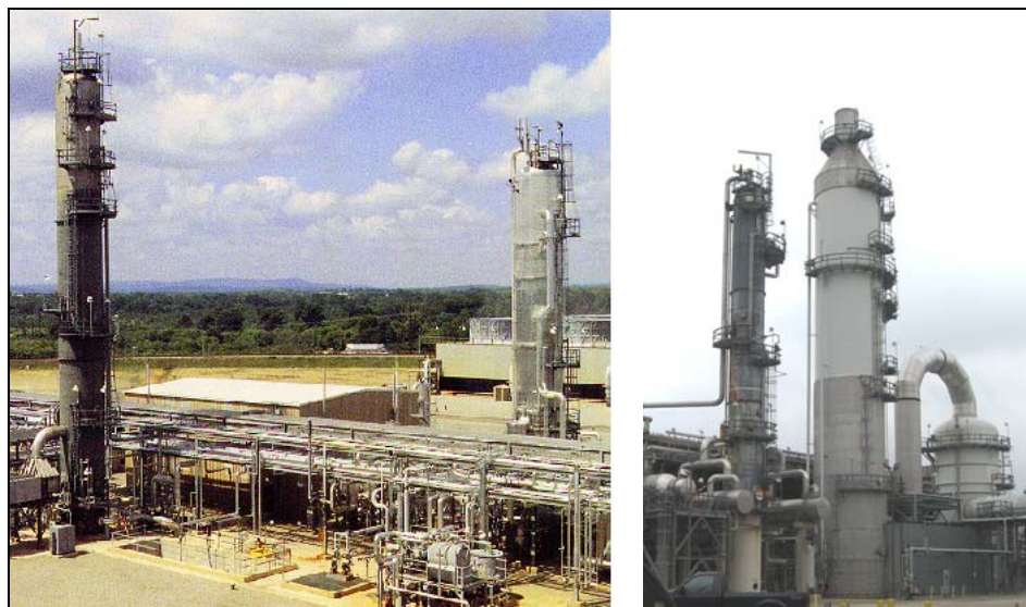
Figure 14. Amine-Based Post-Combustion CO 2 Capture Systems Treating a Portion of the Flue Gas from a Coal-Fired Power Plant in Oklahoma, USA (left), and a Natural Gas Combined Cycle (NGCC) Plant in Massachusetts, USA (right)
