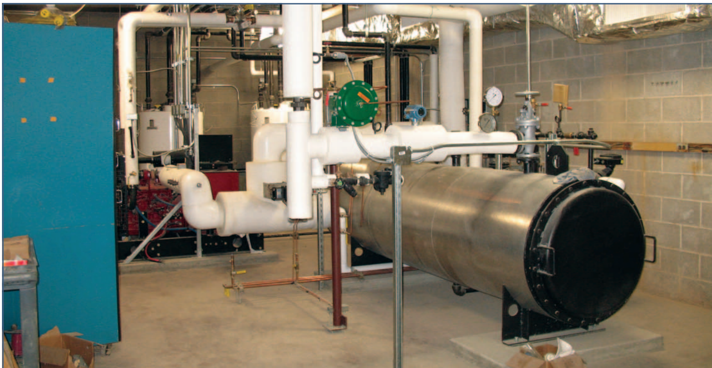
Steam generator in the basement of the Margaret Morrison building.
