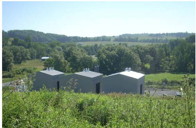
Enclosing compressor stations is a permanent method of noise attenuation. " Gas compressors " by Gerry Dincher, licensed under CC BY-SA 2.0 , cropped from original.
