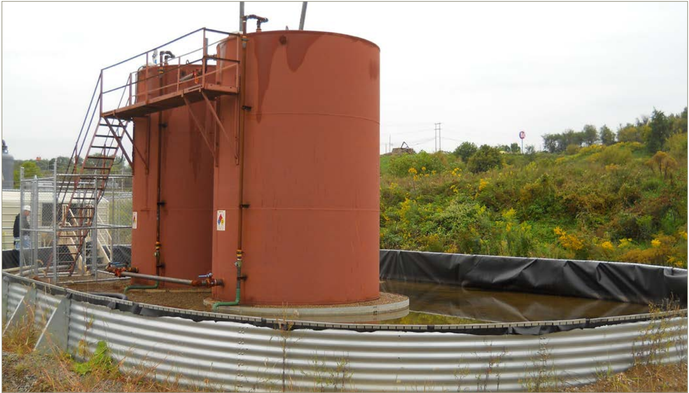
Storage tanks for produced water. " Marcellus Shale Storage Tanks " by Doug Duncan, USGS
