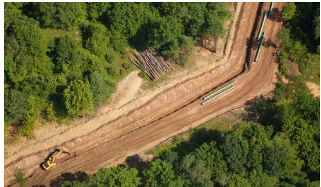
Activities associated with all forms of infrastructure development, including shale gas, such as ground clearing and construction for roads and pipelines (as pictured above), present risks of erosion and sedimentation. © The Nature Conservancy (Mark Godfrey)
