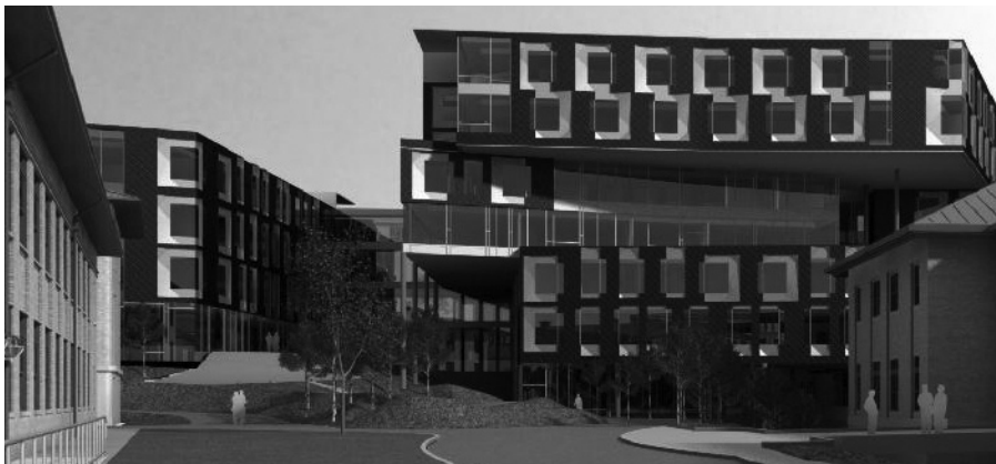
THE GATES COMPLEX, SHOWN HERE BETWEEN SMITH AND NEWELL-SIMON HALLS, WILL INCLUDE 310 PRIVATE OFFICES, 32 LABS, 11 CONFERENCE ROOMS AND A 250-SEAT AUDITORIUM.
