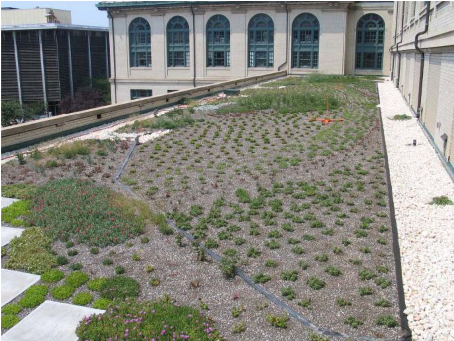
Figure 3: Arching rainbow planting arrangement on the Hamerschlag Hall roof
