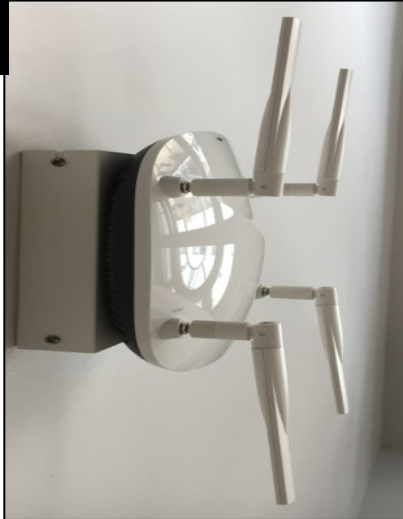
Aruba 324 side view 900 series box mounted on solid surface
